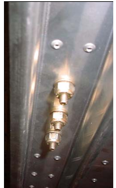
NOTE: The bolts through the Center Bearing 7C4-2 are through the Floor Stiffener 7F8-1
