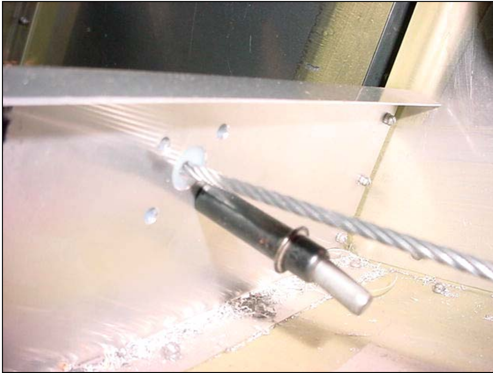
Rudder Cable through a #20 hole in the Fairlead 7C5-6
