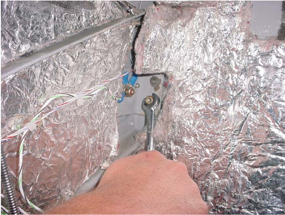
AN3-6A Middle bolt through Steel angle 7F14-5R.
