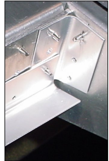
L angle overlaps corner L angle.
