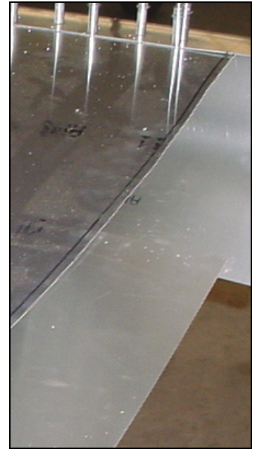
Rough cut the sink approximately 10mm oversize.
